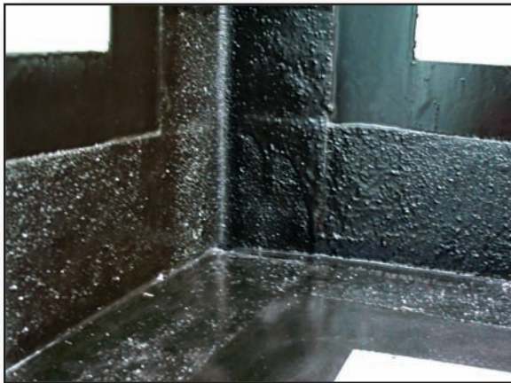
Extra Protection for Leaking Seams
